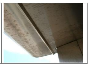
Above is detail of a canopy above a stainless steel revolving door after four years in service in the vicinity of sea water. You can see all kinds of rusty spots also known as tea stains. This is the work of aerosols, together with dirt deposits.
